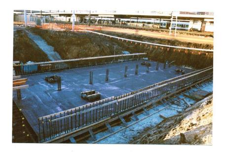
**EVENCURE XDS** hydrocarbon based curing compound being applied to the Spencer Street Subway to Dockland (above) and the Spencer Street Footbridge to Dockland (below) by ASC Pty. Ltd. Evencure XDS is a waterbased product that complies with AS3799 and has the unique ability to oxidise and completely leave the surface within 45-55 days therefore leaving the surface of the concrete in a natural state with minimum preparation for aftertrades.
