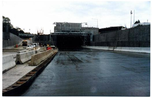
Primecure 90 Bituminous Curing Compound and Primer being applied as a primer on concrete for bituminous overlay by ASC Pty Ltd at the Domain Tunnel, City Link Project, Melbourne.
