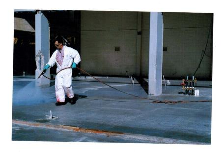
**EVENCURE AC** totally waterbased acrylic modified emulsion being applied by ASC Pty. Ltd., to the Melbourne Grammar Extension on freshly poured concrete. Evencure AC complies the AS3799 standards, dries to a clear finish, will not yellow in sunlight and exhibits excellent durability as a concrete sealer.
