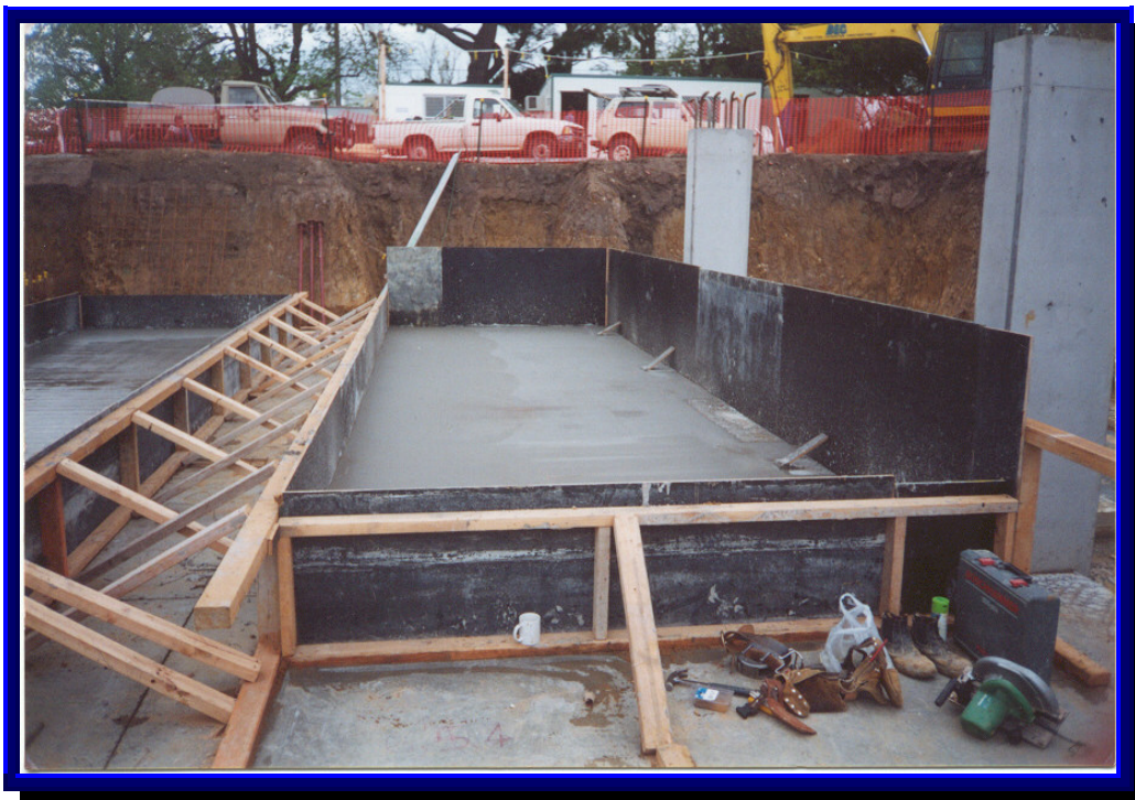
Tilt Slab Wall
